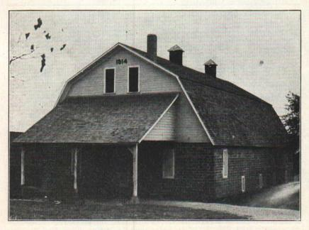
Fig. 2.—One of the older air-cooled storages of the modern type. The size is 36 by 60 feet, including a nine-foot sorting room across the front, and the capacity is about 8,000 bushels. There is an outer wall of eight-inch glazed tile and an inner one four inches thick and between the two is an insulating quilt. The second floor is used for the storage of empty containers.
