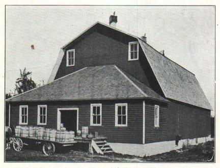
Fig. 1.—This frame storage was built in 1922. It is 40 by 60 feet and has a capacity of 10,000 bushels. A grading room extends across the front. The second floor is used as a storage for empty containers. This is one of the few storages in Michigan with a permanent false floor. A two-inch thickness of hair felt in the walls provides excellent insulation. Note the location of air intakes and outlets.
