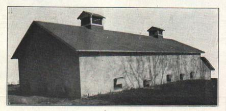
Fig. 3.—The walls of this storage consist of twelve inches of interlocking tile with waterproof plaster on both the inside and outside. It is 33 by 80 feet in size and has a capacity of 12,000 bushels. Hair felt is the principal insulating material of the ceiling. The air intakes are just above the ground line and are well distributed about the building. The air outlets are each 4 by 4½ feet.
