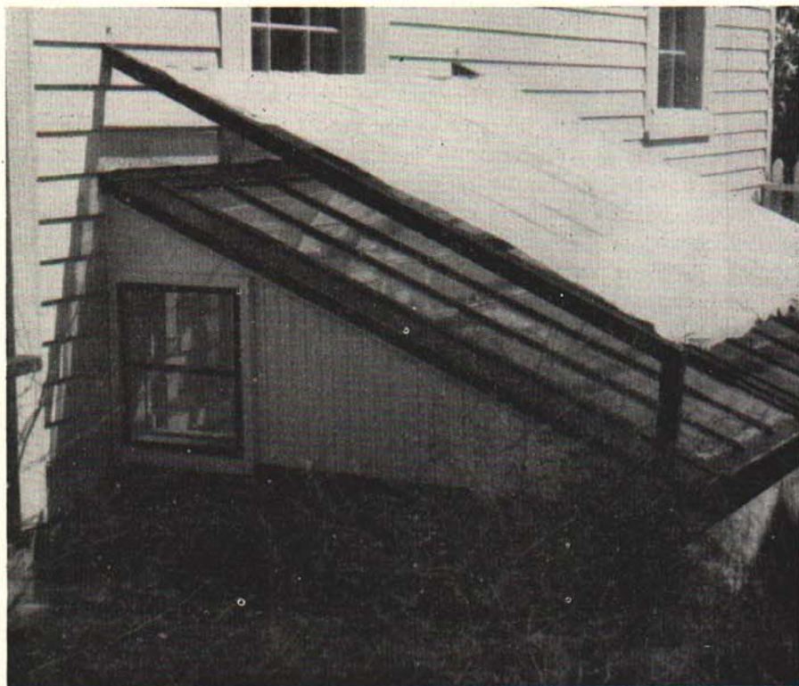
Fig. 2. A hotbed heated through a basement window.
