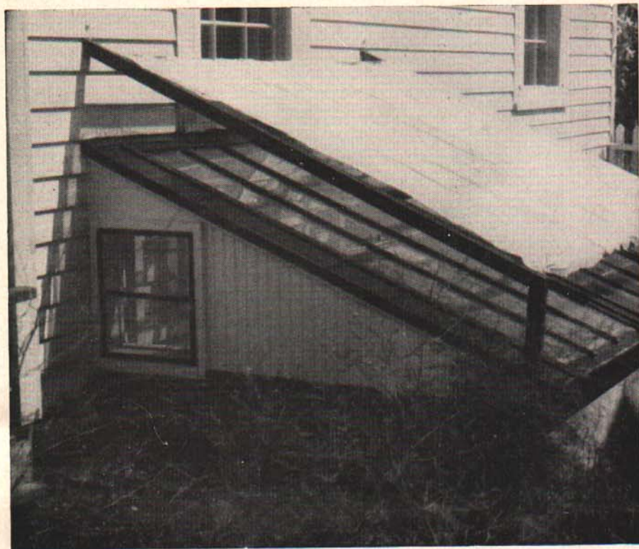
Fig. 4. A hotbed heated through a basement window.
