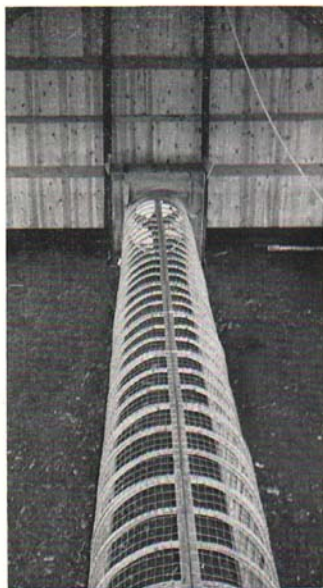
FIG. 7.—Commercially made steel duct.
