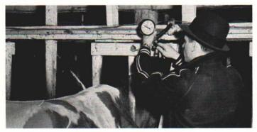
Fig. 6. Checking the vacuum pressure is necessary to maintain proper milking machine operation.
