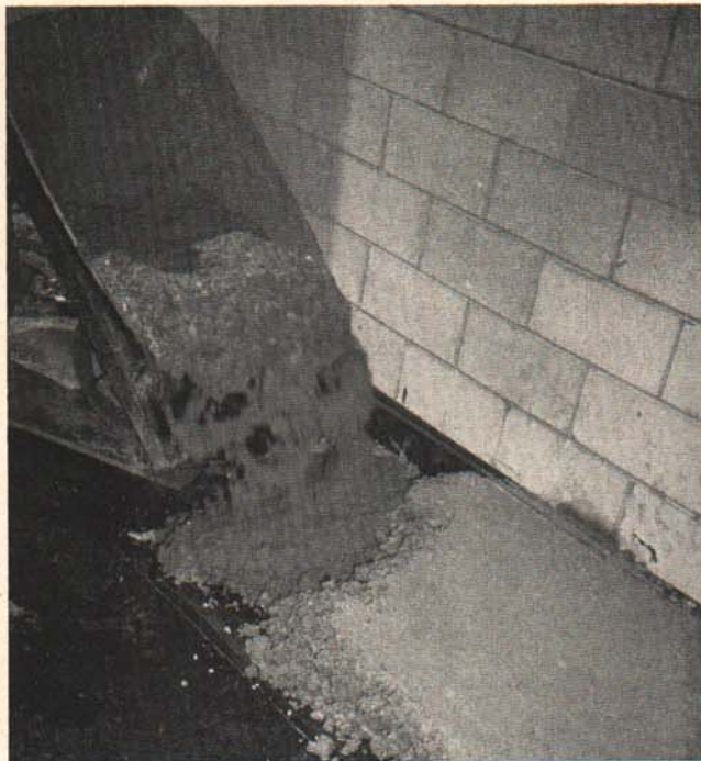
Fig. 13. Pouring the finish coat. Concrete should not be poured from a height greater than 4 feet without a chute.
