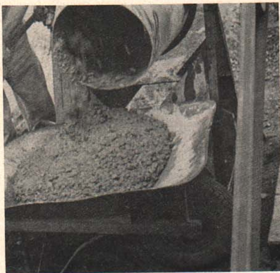
Fig. 7. A well-proportioned concrete mix.
