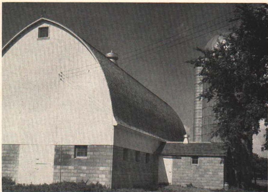
Fig. 23. A two-story dairy barn with an attached milkhouse of concrete masonry.
