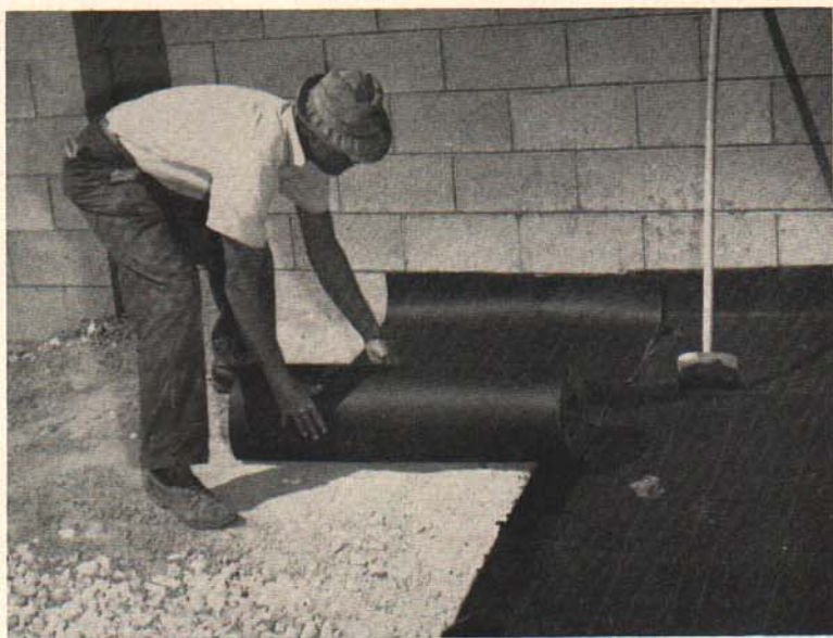
Fig. 12. Laying the vapor barrier for a moisture-proof floor.
