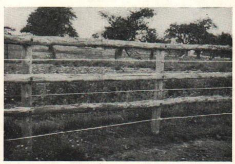
Fig. 6. Electrified wires reinforce aging pole fence. Note—Even with new strong poles, the wires are desirable if but three poles are used.
