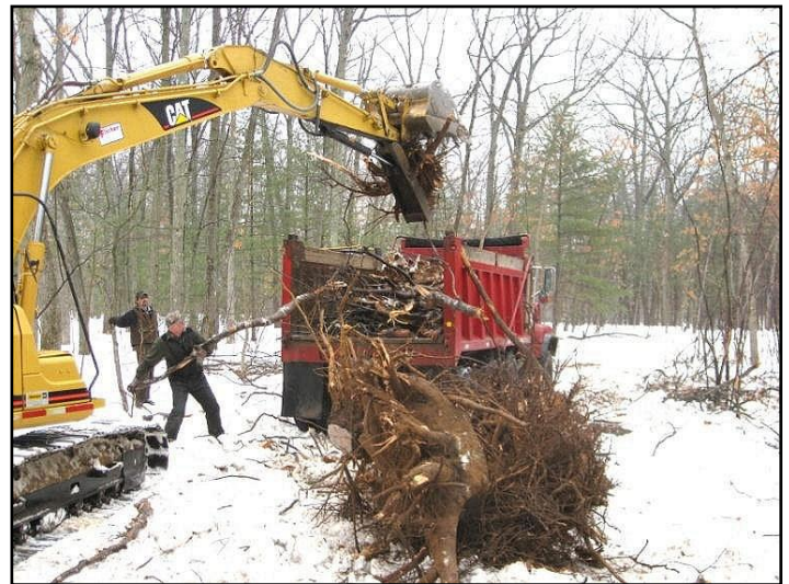
Figure 21. Stump-pulling and chipping.
