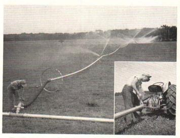
Fig. 10. Two types of labor-saving irrigation equipment, which simplify the moving of lateral lines. Both use flexible hose couplings for quick re-attaching to main line valves. A ratchet drive allows one man to roll a 40-rod lateral into position in the "wheel move" system. In a "tractor tow" system (inset), the entire length of the lateral is simply snaked across the field.
