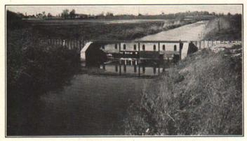
Fig. 1. Dam constructed to maintain water level in a large muck area. Note the use of interlocking sheet steel piling, which is driven deep to extend well out into the bank on each side. It is also driven across the ditch below the bottom of the gates. Concrete piers, concrete apron in the bottom of the ditch, angle iron braces welded into position, and four redwood gates complete the construction.
