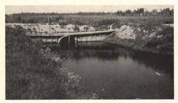
Fig. 4. View of secondary dam and bridge in the Chandlers Marsh drain, nine-tenths of a mile above the master dam shown in Fig. 3. This photograph was taken from the upper side, in late summer, before the retaining planks had been removed to lower the water level.
