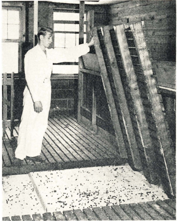
Fig. 5. Slatted flooring hinged at the base. The sections can be raised to clean them. Note the gutter in the left foreground.
