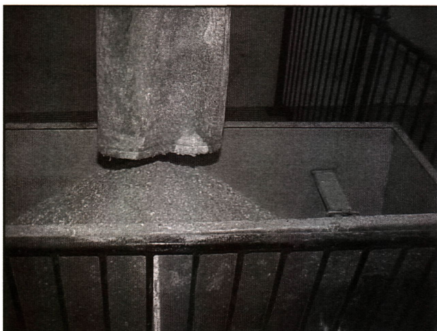
Figure 2. Placing covers over feed drop spouts can reduce dust.
