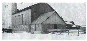
Fig. 3. Concrete blocks make an excellent first-floor wall for remodeled barns.
