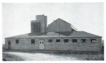
Fig. 7. Single-story dairy barns of concrete block construction are fire-resistant and serviceable.
