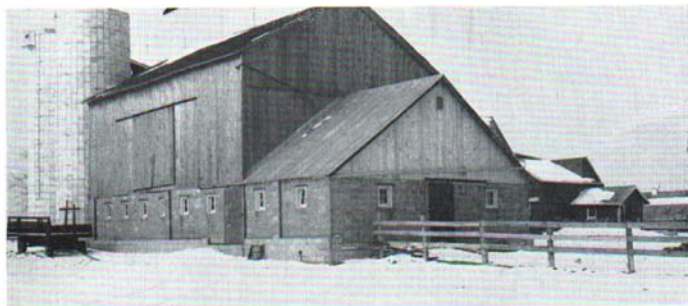
Fig. 3. Concrete blocks make an excellent first-floor wall for remodeled barns.
