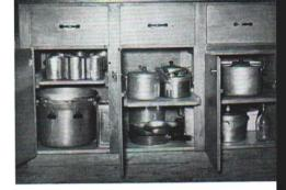
In this cupboard the shelves have been spaced to fit the utensils to be stored. Notice that the top shelves can be pulled out when utensils are placed in or removed from cupboard. This type of shelf is very desirable for the lower cupboard.
