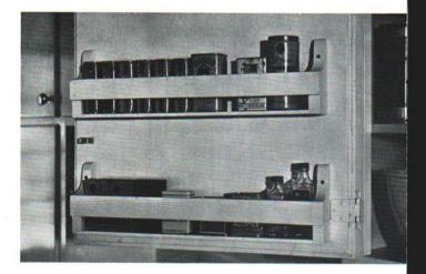
Racks for spices, extracts, etc. can be fastened to most every cupboard door. The length of the rack is determined by width of door. The depth of rack should depend upon the size of cans or items to be stored. The bar or strip across front of rack should be placed about one inch from the bottom and so it does not cover the names on cans.
