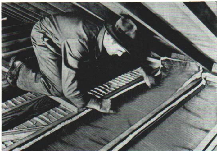
Fig. 4. Installing a flexible insulating blanket between floor joists in an unfinished attic.
