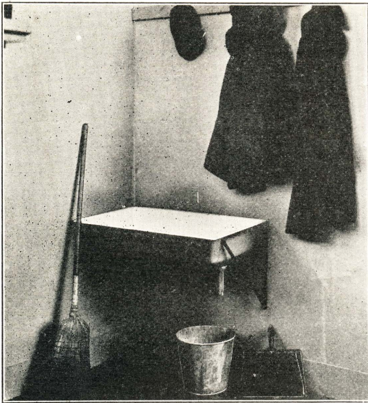
Figure 1: A sink improperly located with an inadequate method of sewage disposal. It is of little value.
