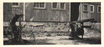
Fig. 7. Power, clutch and shaft arrangement of a dairy barn where one motor and a gear reduction unit operate both aprons of a two-gutter, face-in-type barn. The clutches are grab type. (George Bailey farm in Hillsdale County.)
