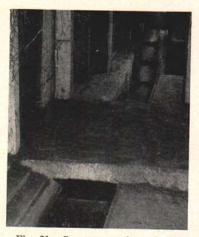
Fig. 21. Over-pass at the end. Note grooves on the top of the gutter for cover plates. Elevator and drive shaft in background.
