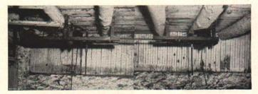
Fig. 8. The interior view of a dairy barn, showing the apron-return arrangement using one motor to operate two drums. Clutches are friction-disk type.
