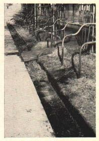
Fig. 5. The interior view of the A. J. Cable dairy barn, showing the single gutter and the return cable on the lower end. Note how clean the gutter is left as the apron moves out.
