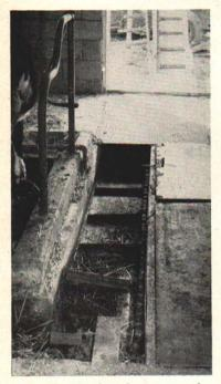
Fig. 17. Part of metal cover removed to show details of slats turning on themselves.
