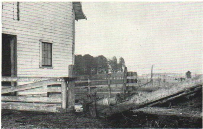
Fig. 6. On barns where the gutter cleaner must be installed in the same end of the barn as the hay barn door, the gutter may be extended 14 to 16 feet to permit a drive near the end of the barn. This picture shows the installation on the Dale Woolcott farm in Van Buren County.
