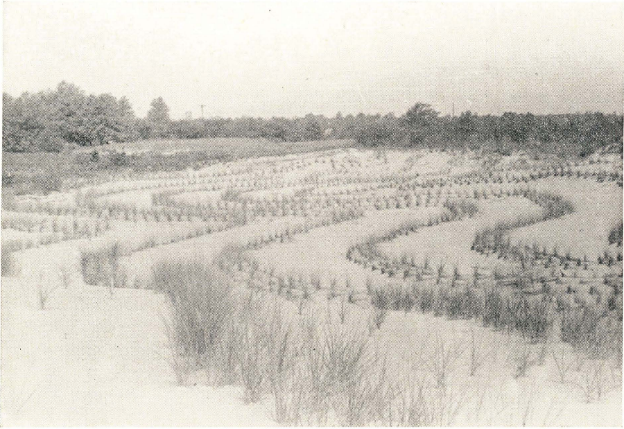
Fig. 2. Temporary stabilization of blow sand by planting curving rows of beach grass.
