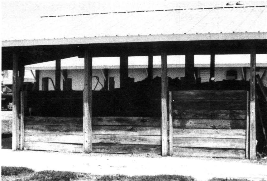
Figure 1. Unit for composting dead pigs. Each of the six bins is 5 feet tall, 8 feet wide and 5 feet deep. A facility of this size would accommodate a typical 100 sow farrow-to-finish operation.
