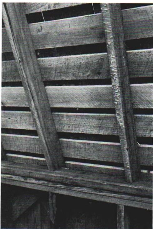
Fig. 13. An excellent roof deck, using sound uniformly sawed roof boards, properly spaced for nailing shingles. This construction is preferable to that shown in Fig. 14.
