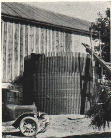
Fig. 1. A well built crib silo, showing details of construction.
