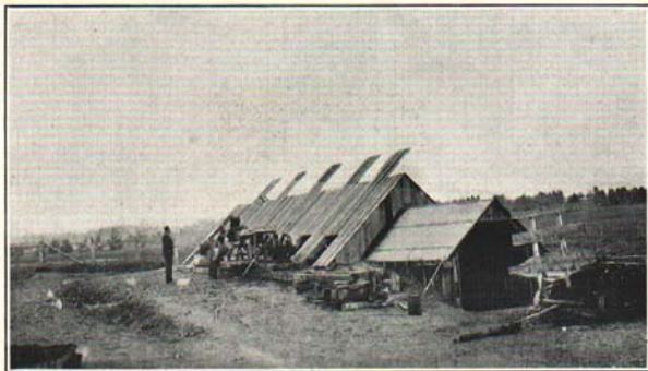
Fig. 8. Using low-cost machinery for filling.
