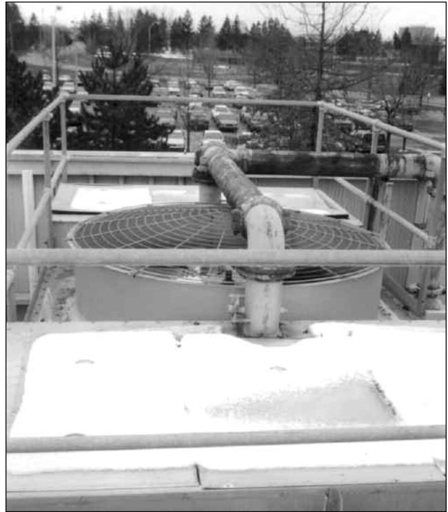
Removable sunlight covers on distribution decks are used to minimize algae growth. (Winter photo shows snow on covers.)
