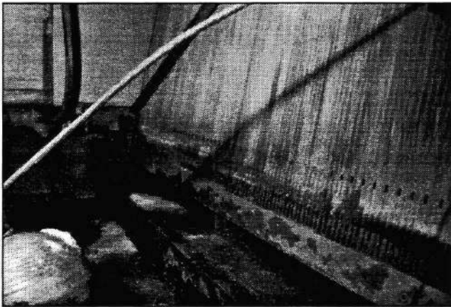
Inside the basin of cooling towers there are many surfaces and areas that provide favorable places for microbial organisms to grow.
