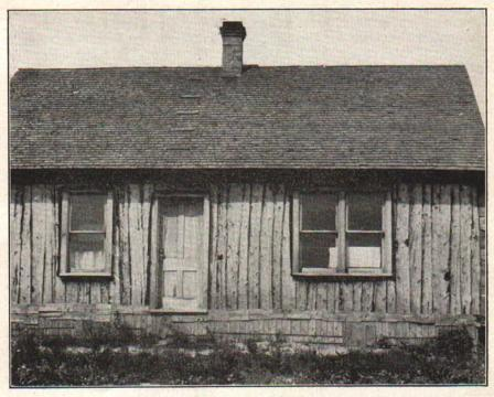
Fig. 8.-A house made of cedar logs, hewn and set on end.
