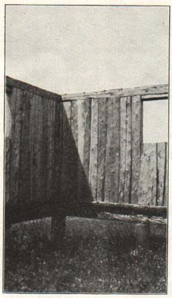
Fig. 12.—A barn basement being built of cedar logs set on end. The method of nailing them at the top and bottom between two long logs is clear. This type of basement was used in the barns shown in Figs. 17 and 18.
