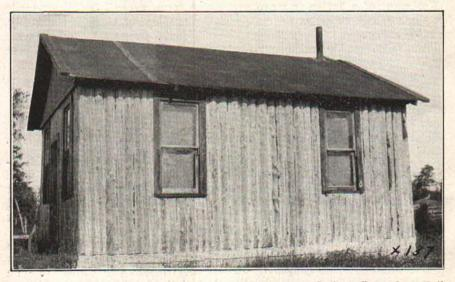
Fig. 9.—A pole house makes a comfortable temporary home. It is easily made, and the poles can be cut on the farm, saving time and hauling expense. Smaller poles were used in this house than those shown in Fig. 8.
