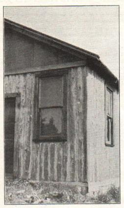
Fig. 10.—A corner of the house in Fig. 9, showing how the poles are set and matched.
