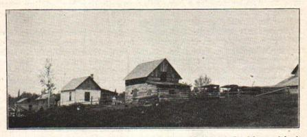
Fig. 4.—A complete set of farm buildings near Republic, Michigan, built of logs and lumber sawed on the farm. The cost of these buildings, not counting the owner's labor, was about \$450 A better arrangement of the buildings would have added to the convenience of the farm and made possible better use of the log houses when permanent buildings were erected.
