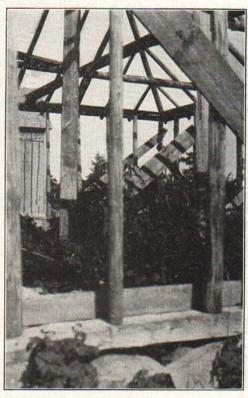
Fig. 6.—A corner of framework made from spruce and tamarack poles. The poles are toenalled to the hewn log used for a sill.
