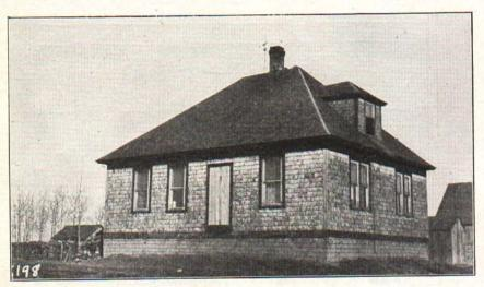
Fig. 14.—This house was made of cedar logs, as was the house in Fig. 8. The logs were then covered with shingles, making a neat and weatherproof home.
