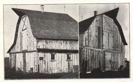
Figs. 15 and 16.—Showing how the barn (started as illustrated in Figs. 12 and 13) was finished, with poles for frames, and covered with lumber that was sawed from logs taken from the farm.
