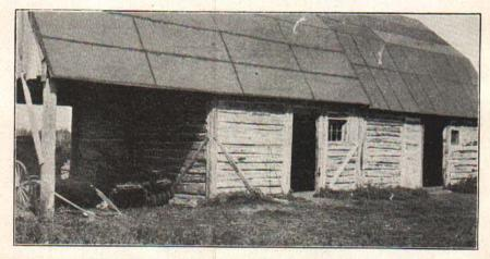
Fig. 19.—Barn made of cedar logs laid horizontally. It would have been better if more windows had been provided. The ends are toenalled to corner logs, instead of the method of notching and crossing used in other log buildings.
