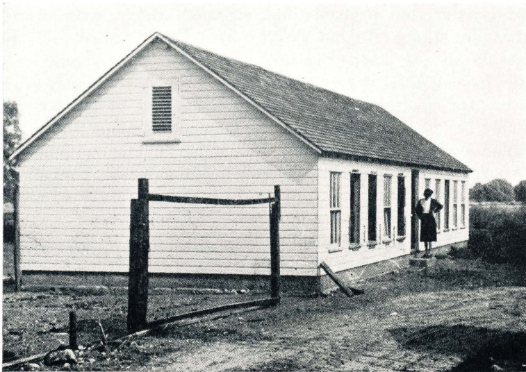
Fig. 12. A gable-type 20' x 40' straw loft house.
