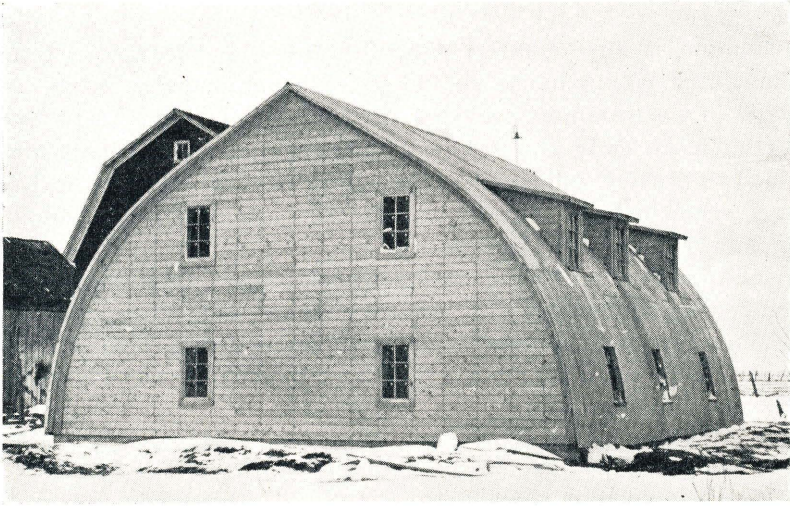
Fig. 2. A southwest view of the 36' x 36' two-story laminated-rafter type laying house. The stairs to the second story are on the east side of the building.
