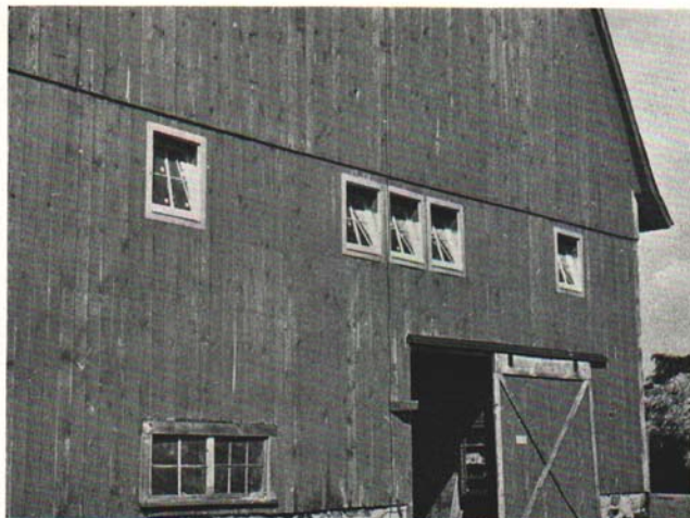
Fig. 17. Changing the hay mow over into a laying house. Note the use of galvanized window sash, which eliminates much labor in the framing of the window.
