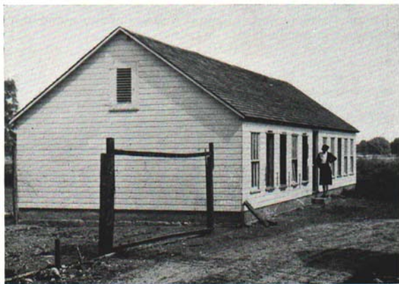
Fig. 12. A gable-type 20' x 40' straw loft house.
