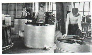
Fig. 28. Extracting equipment. Note "wing" comb supports in first extractor. Note arrangement, comb tables near each extractor, honey piped through floor, motors mounted above extractors with V-belts, ample room to truck empty supers on platforms away from extractors.
