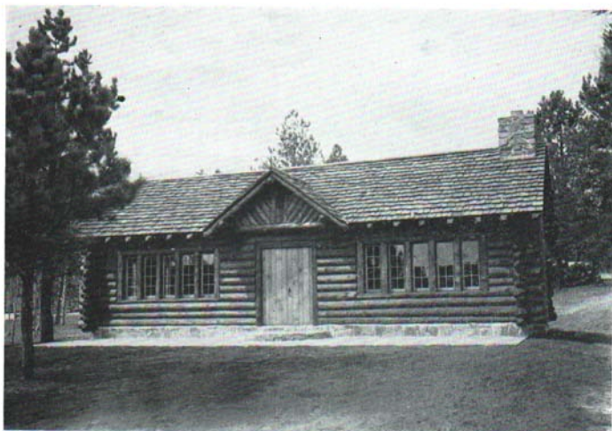
Fig. 5. A well-constructed, well-lighted cabin suitable as a small school house. Heavier hardware for the door would have been more appropriate. (Photograph by the U. S. Forest Service.)
