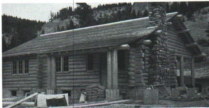
Fig. 14. Attractive log work in a U. S. Forest Service ranger station. The structure features a full basement and ample porch space. It might have been much more attractive had the foundation been constructed of material similar to the fireplace.
