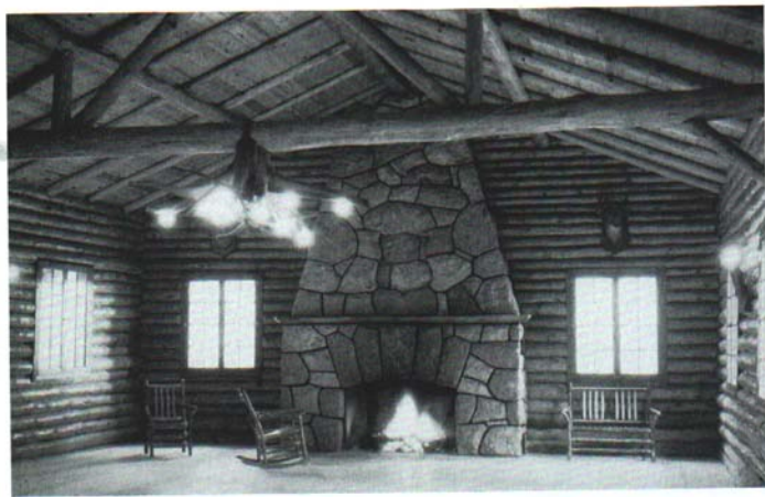
Fig. 17. A cut-rock, circulating fireplace. Registers are on the side. Individual rocks have been accentuated with an outline of black mortar.
