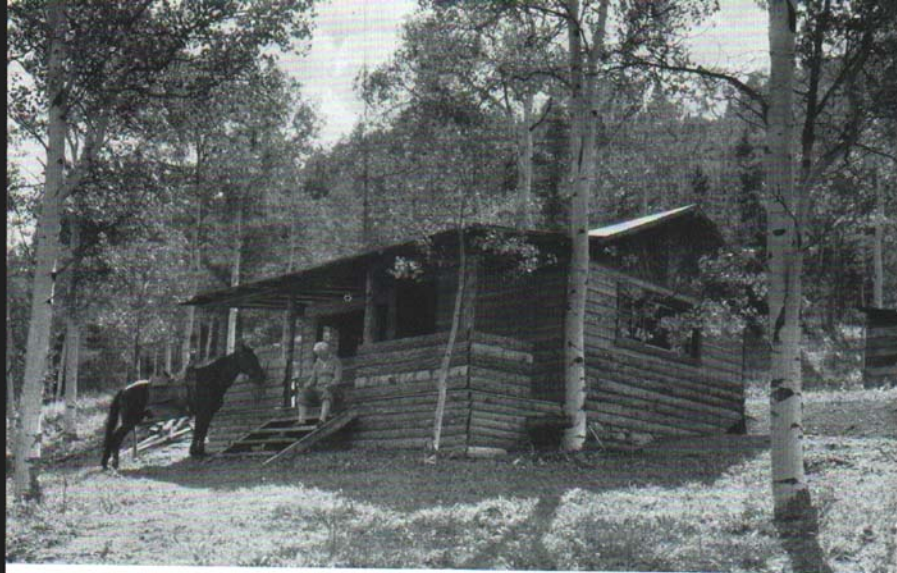
Fig. 12. Ordinary beveled siding has been used in this cabin to accentuate the door and window framing. Exclusive use of slabs would not have produced the same effect. The owner obviously has failed to protect the woodwork against decay organisms inasmuch as the rear portion of the cabin is resting directly on the ground and permits no aeration under the floor. (Photograph by U. S. Forest Service.)
