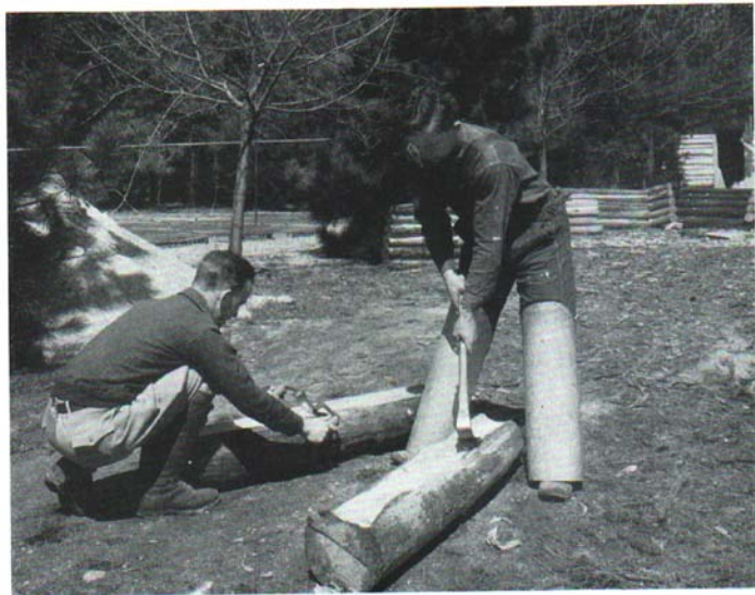
Fig. 8a. Cutting grooves with curved adz and draw knife.
