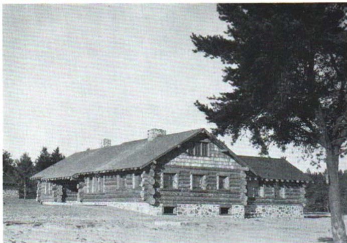
Fig. 6. A pleasing combination of materials distinguishing floor levels. Note the precautions taken to aerate the timbers beneath the main floor. (Photograph by Michigan Dept. of Conservation.)
