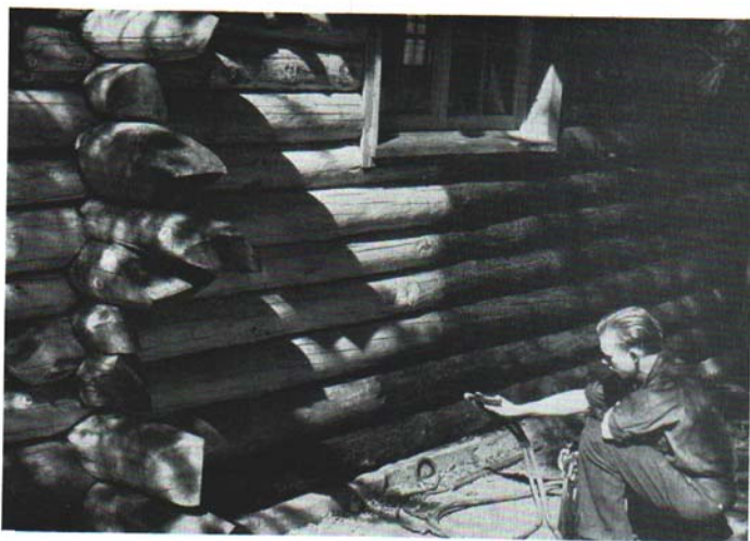
Fig. 25. Treating the exterior with a creosote stain.
