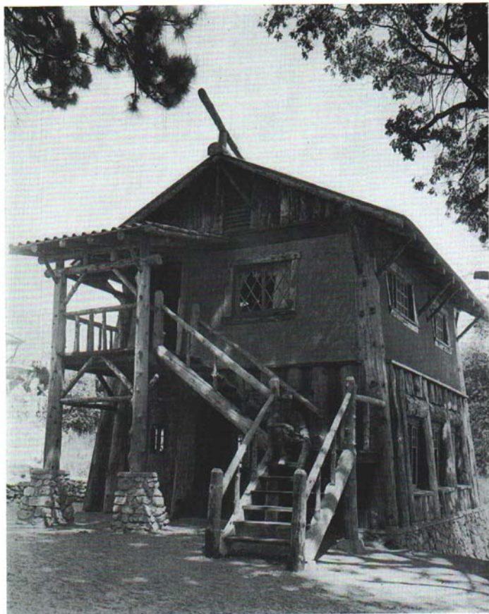
Fig. 2. An unusual design bordering on the ornate. The selection of tin roofing and stucco to accompany the rather attractive log work has largely destroyed the finer characteristics of the cabin. (Photograph by the U. S. Forest Service.)
