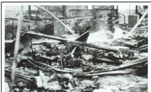
Figure 1. A majority of all farm fire losses are related to electrical system failure.
