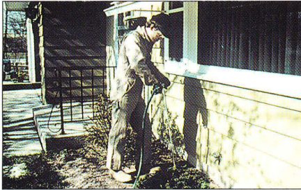
Long rodding exterior of house
