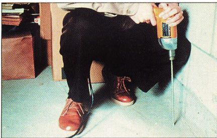
Drilling a slab
