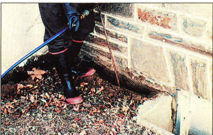
Rodding and trenching basement
