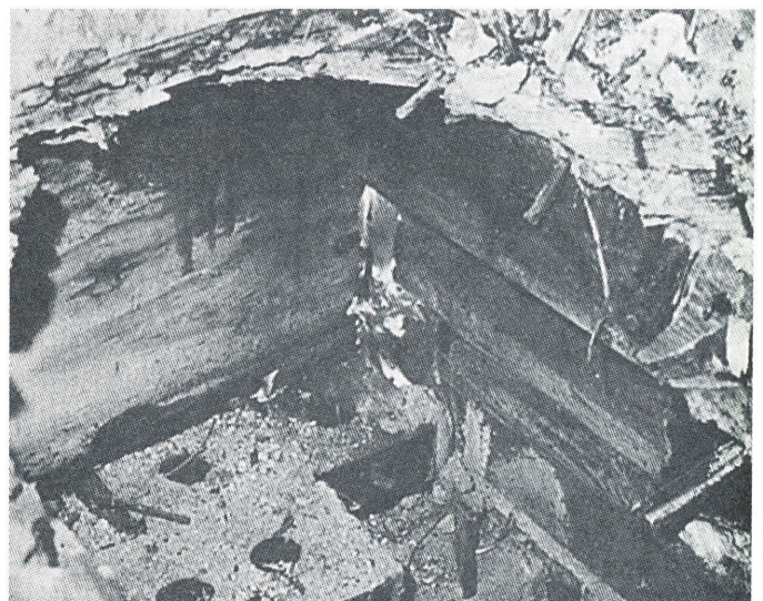
Figure 7.3. Rhizomorphs of Poria growing from earth-filled porch.
