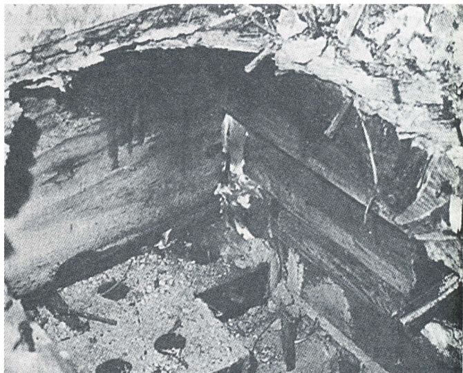
Figure 7.3. Rhizomorphs of Poria growing from earth-filled porch.
