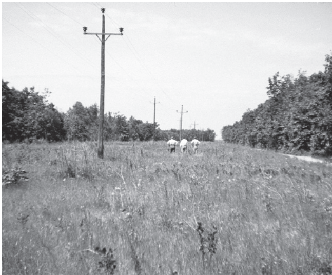
Examine the site to identify site specific requirements.
