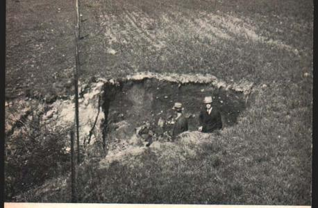
Fig. 17. The brush on the left piled in this gully failed to stop its growth into the next field to the right of the fence. Gullies are stopped by diverting water into new channels further up the slope. Grass, cover crops, contour cultivation and diversion of water by terraces or other means are necessary to prevent formation and growth of gullies.
