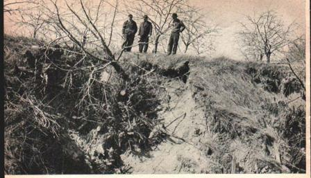
Fig. 10. One of three gullies doing serious damage in a valuable orchard. The owner is asking the county agricultural agent and a representative of the Soil Conservation Service to suggest means of control.
