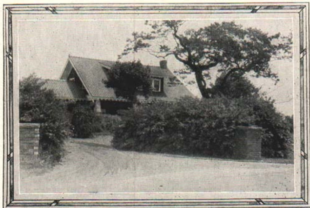
Fig. 20. A simple, dignified, and pleasing entrance drive.
