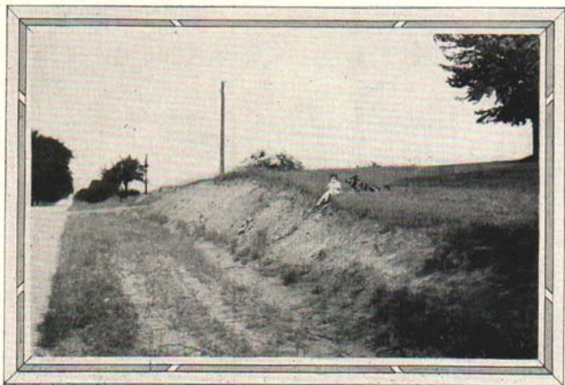
Fig. 17. Before grading. Steep roadside banks are displeasing features in informal landscape developments. (See Fig. 18.)
