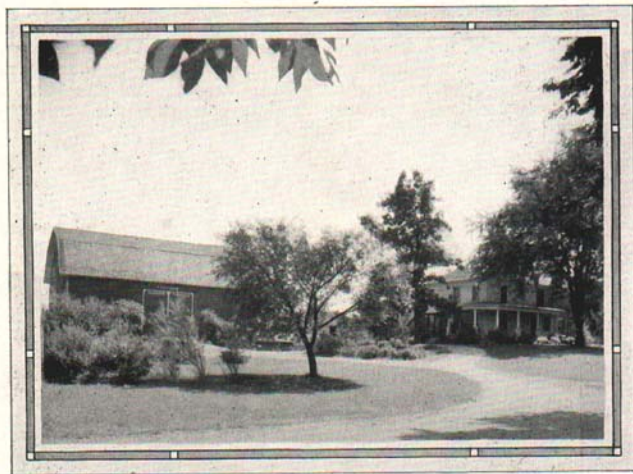
Fig. 21. Entrance to the home grounds showing the "turn-around" drive See design of drive, Fig. 6.
