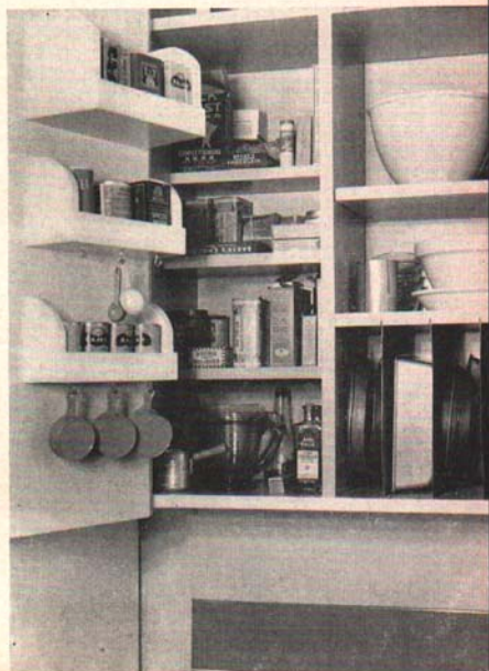
Fig. 7. This cupboard is placed next to the refrigerator, and a few steps from the sink. The doors are hinged so that the entire cupboard opens wide to leave everything accessible. Here are stored the staple foods and equipment necessary when such foods as a cake or biscuits are to be mixed. Notice the racks on the door (graduated in size) for storing spices, and the removable vertical partitions in the lower righthand shelf for storing pie-pans and cakepans.
