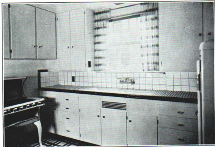
Fig. 21. A compact convenient kitchen arrangement. Notice these features: light in ceiling above sink, wall outlets for small electrical equipment, cupboards on wall space over the range, glazed tile working surface, double sink, ventilated cupboard below sink, and toe space at bottom of cupboard.
