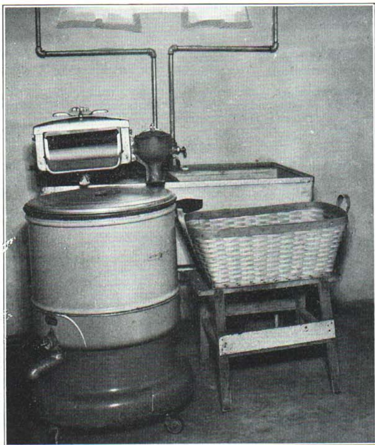
Fig. 2. Convenient arrangement of washing equipment including machine, two stationary tubs, basket and stand. The tubs are equipped with hot and cold water and drains.
