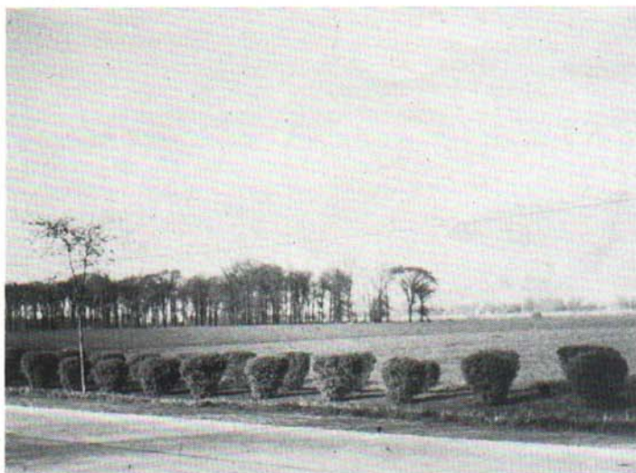
Fig. 13. A mass planting of shrubs along highway improperly pruned.
