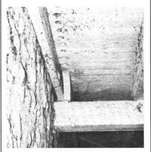
Figure 15. Three-inch diameter holes drilled in a ceiling to approximate a slot inlet.
