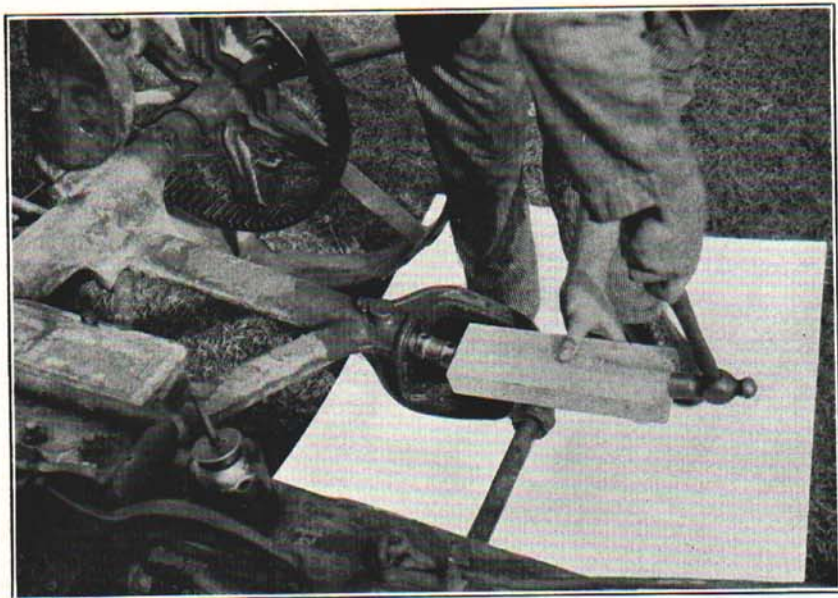
Fig. 7. Replacing lower crankshaft bearing. Fly-wheel removed.
