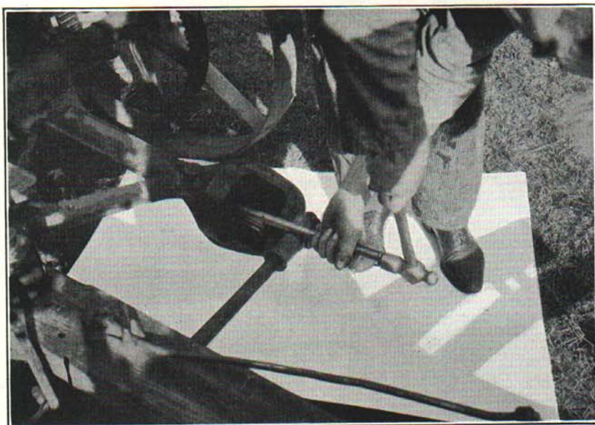
Fig. 8. Removing fly-wheel.
