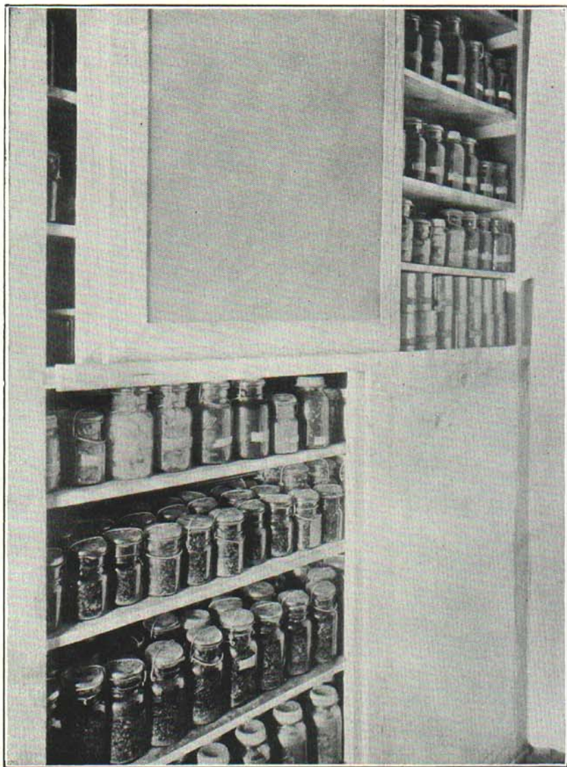
Fig. 19. The arrangement pictured here for the storage of canned products protects them from light and dust by the addition of sliding doors to the shelves. If the groove is kept waxed the doors slide easily and do not require floor space when being opened.
