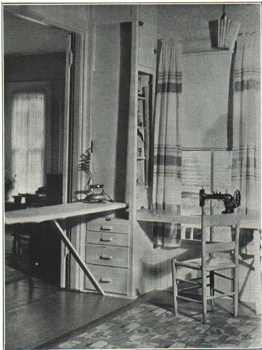
Fig. 23. The combination of the ironing and sewing center has many advantages. Behind the ironing board are shelves for storing sewing supplies. The drawers below the ironing board can be used for sewing and ironing equipment. The electric sewing machine is placed in a hinged shelf. When the machine is not in use it can be removed and stored away and the shelf fastened up on the wall. This shelf would also be convenient for stacking clothes or holding the clothes basket when ironing. This unit has good light and ventilation, which are important for such a center.
