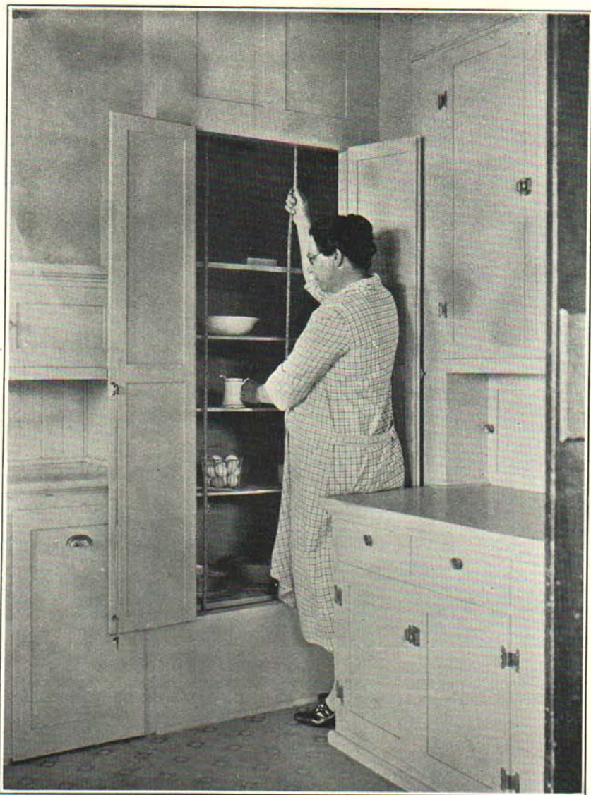
Fig. 16. A dumb waiter such as the one pictured here saves many steps to the basement and is a satisfactory substitute for a refrigerator except during the extreme hot weather. It should be built so it is easily pulled up and can be securely fastened into position.
