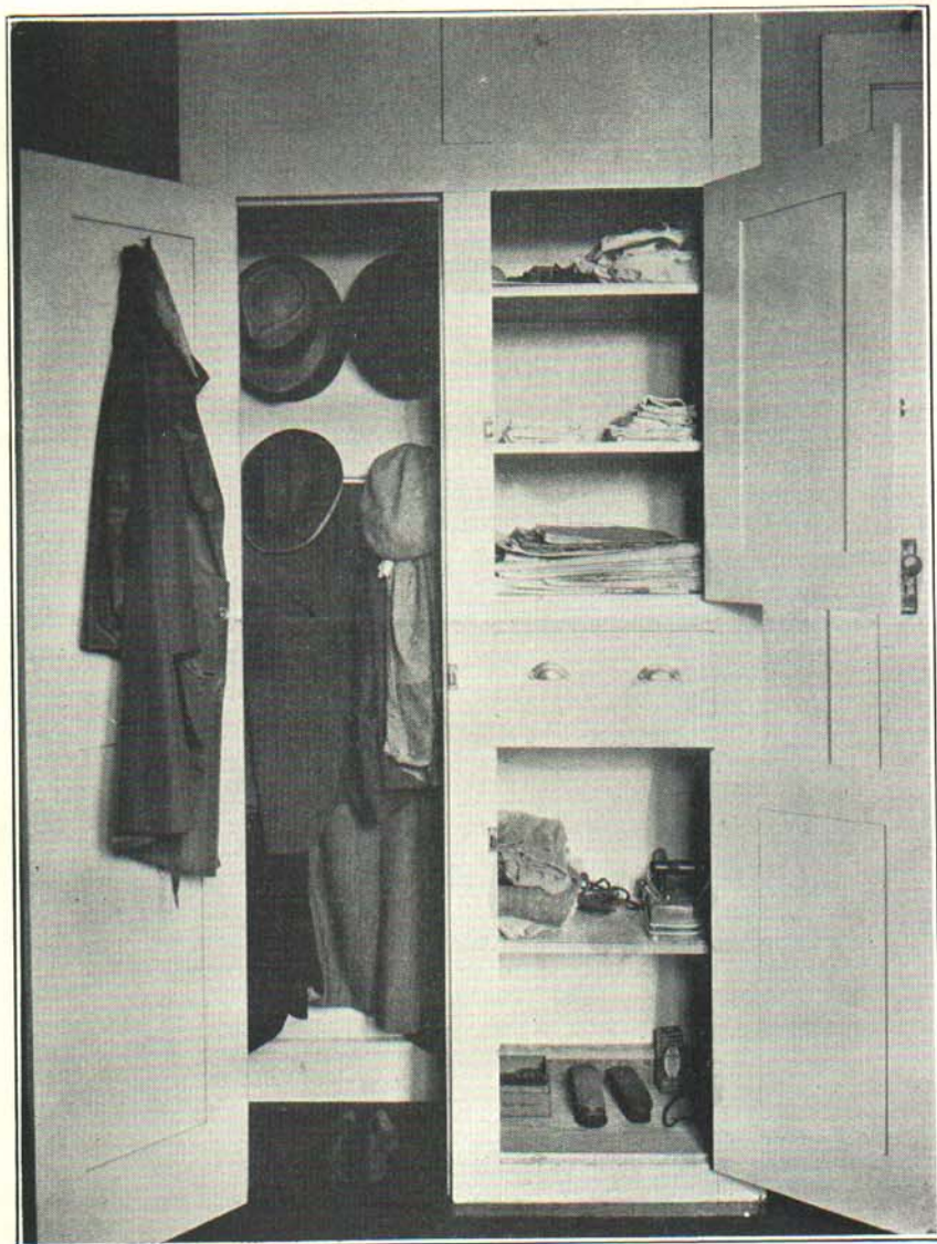
Fig. 1. A cupboard and closet of this type can be built in the kitchen, hall, or back entry for the storing of every day wraps. The shelves and drawers are used for miscellaneous storage. The shelves and drawers the entire lower section used for hanging the children's clothing. A rack for rubbers and overshoes could then be built into the back of the full length cupboard. The size depends upon space available.
