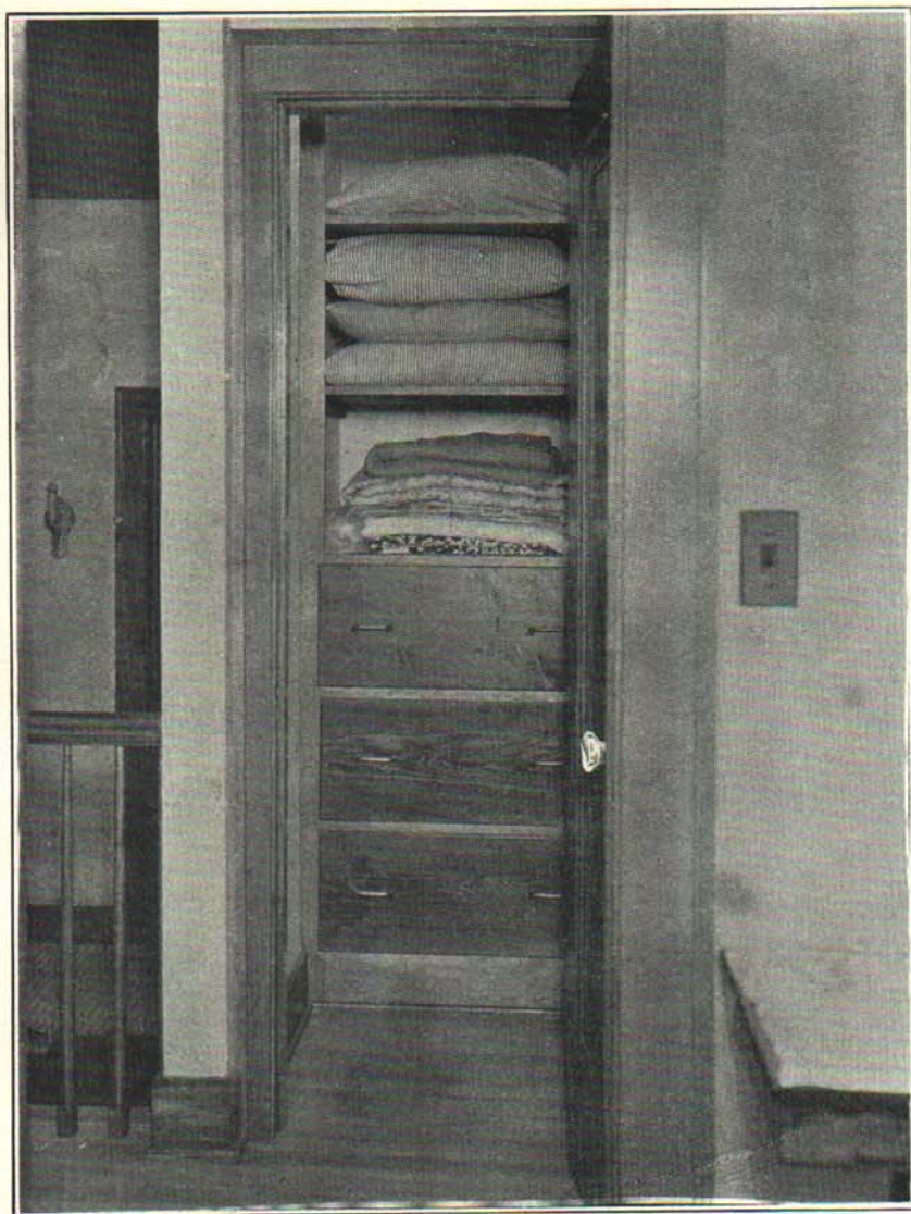
Fig. 10. A linen and bedding closet conveniently located in the central hallway of the second floor. The broad deep shelves and drawers are particularly convenient for storing bulky articles. There is a ceiling light fixture which operates by a pull cord.
