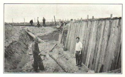
Fig. 4. A trench silo under construction in the Upper Peninsula.
