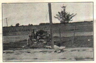
Fig. 15.—A piston pump operated with an electric motor pumping from 4 shallow wells.
