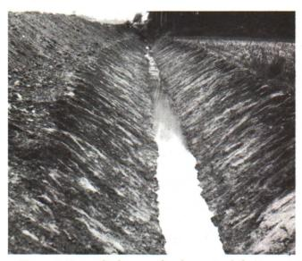
Figure 7. Open ditches can be dry part of the year or contain water. Engineers should design open ditch systems, but ideally, crop producers should maintain them. Seed grass to stabilize sides of ditch so that sedimentation does not reduce ditch depth.
