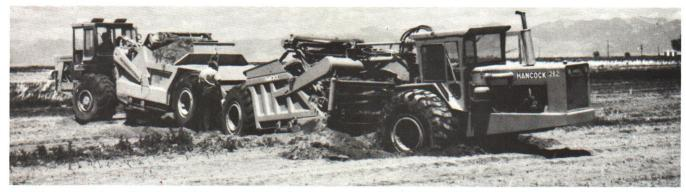
Figure 2. Land grading is a job for professionals. Here, an earthmover got stuck while preparing a field for surface drainage because the soil conditions were not correctly evaluated. Land grading should be used in Michigan with caution because surface soil layers are usually thin. Soil physical and chemical problems are common when subsoil is exposed.
