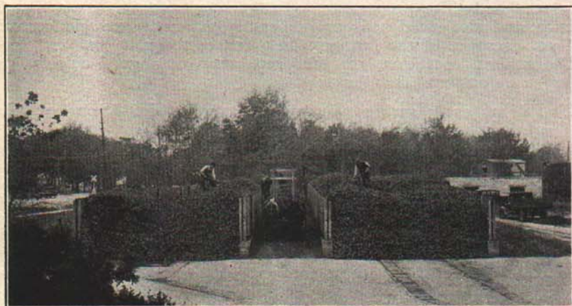
Fig. 4.—Delivery of chicory into storage bins. In the foreground are the flumes through which the roots are floated into the washer and cutter. The cut roots are then elevated to the top of a high building to begin the drying process.
