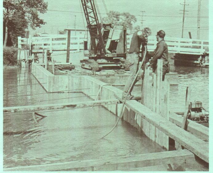
Fig. 1. Retaining walls along waterways need preserved wood.
