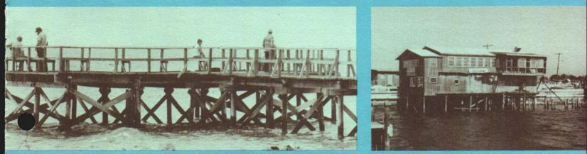
Fig. 15. (Left) Fishing piers are commonly made with salt-treated decks and creosoted or PCP-treated piling in fresh water. Fig. 16. (Right) Buildings such as this restaurant are supported on treated piles.
