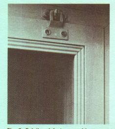
Fig. 5. Painting defects caused by excess absorption of preservative by screen sash.
