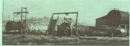
Fig. 7. Three treating cylinders used for full cell or empty cell pressure treating.
