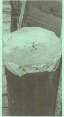
Fig. 9. (Left) Deterioration of unprotected pile. Fig. 10 (Above) Metal cap to protect piling. If metal is broken, water can enter and protection is reduced. Coal tar pitch or grease preservatives also can be used.
